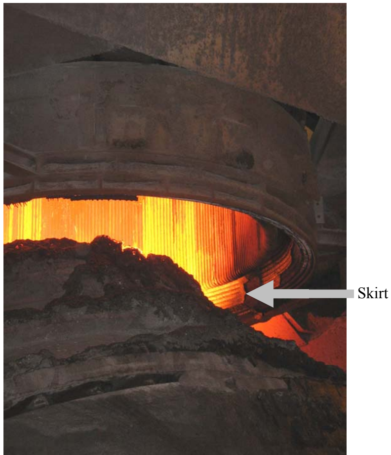
Figure 2. Aluminum Bronze Skirt Installed
